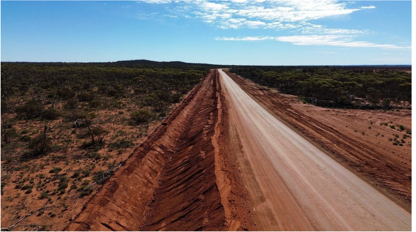
Plate 3 TSF/Hall Road drain.
