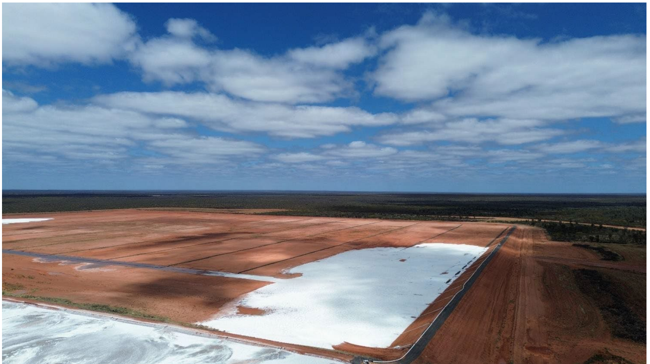
Plate 1 TSF Cell 4 Pipelines installation.
