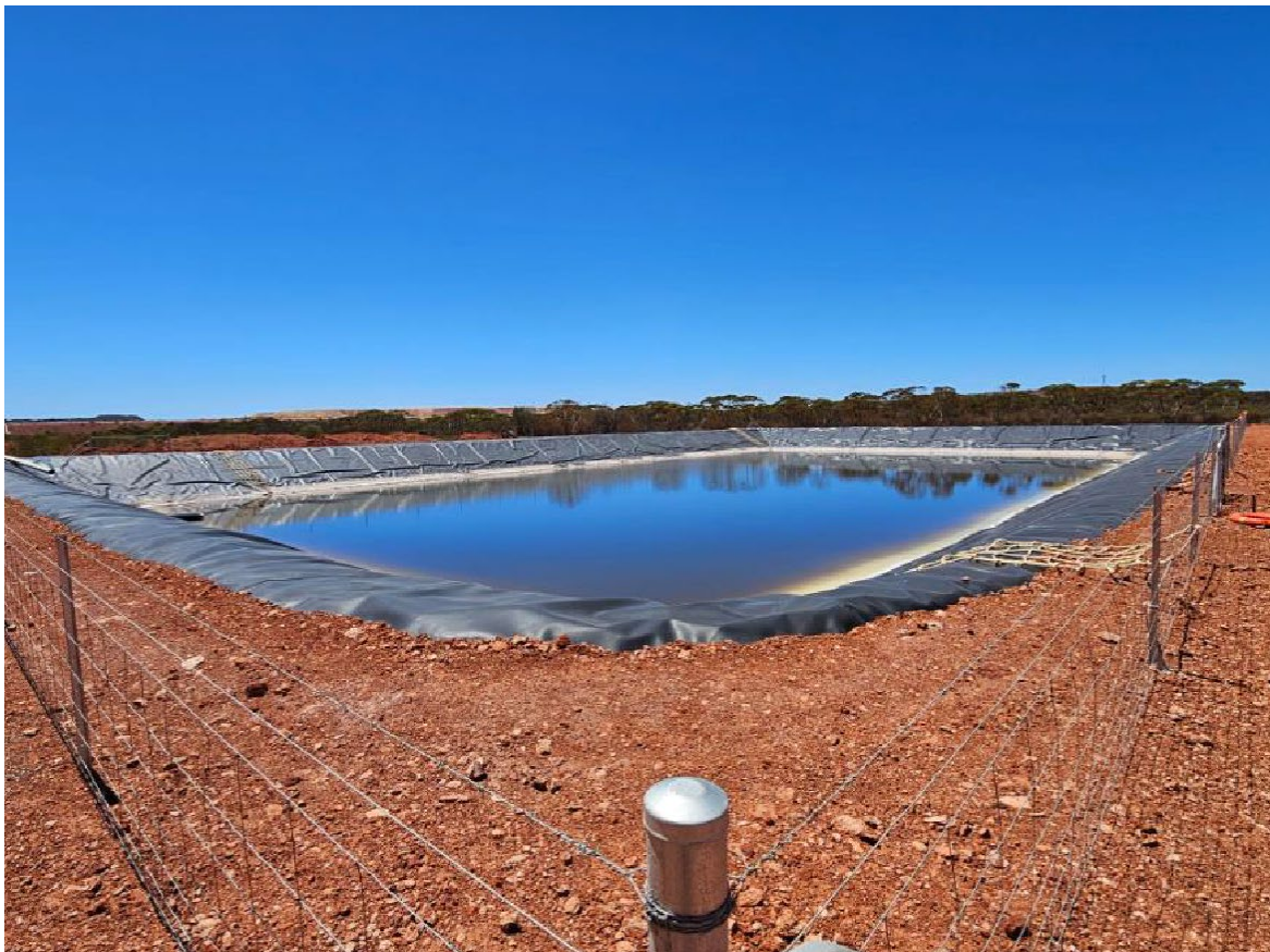
Plate 6 Fencing and Fauna egress netting around water holding facility.
