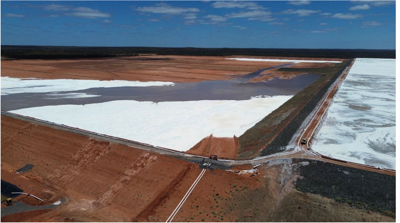
Plate 4 TSF Cell 4 - Commencement of Tailings discharge.
