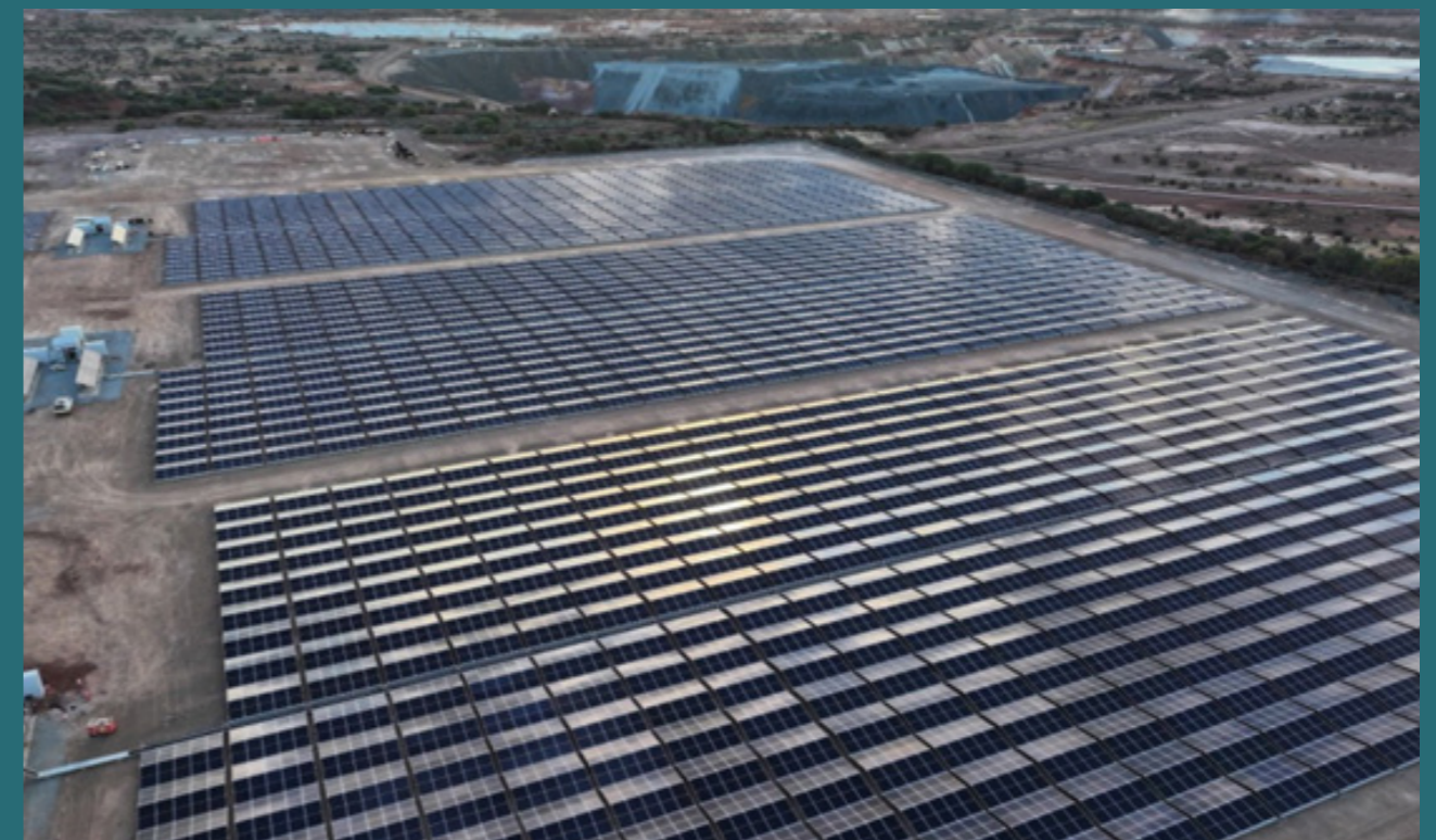
Figure 4 Completed solar farm at Jundee Operations
