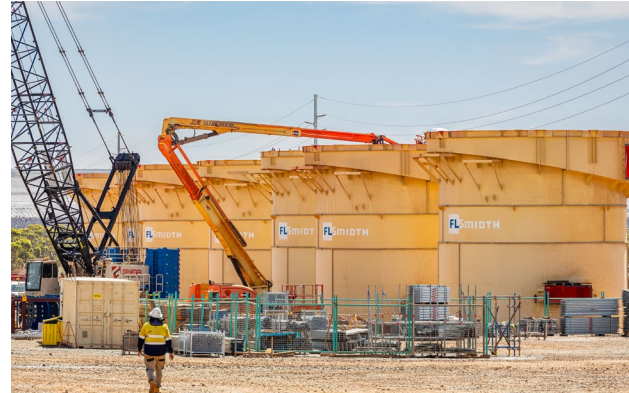
4. Flotation Cells Ready For Installation
