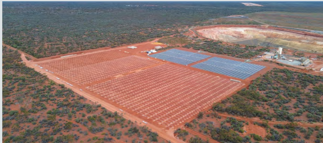
Figure 5 Clearing has been completed for the new 8MW solar plant at Carosue Dam Operations (existing solar farm adjacent)
