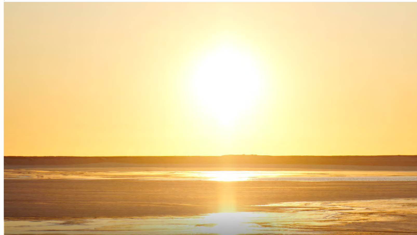
Sun setting over our Thunderbox Operations TSF Thunderbox Operations, Yandal Production Centre, Western Australia
