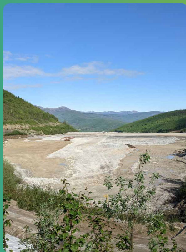
Dry stack tailings facility at Pogo, Alaska
